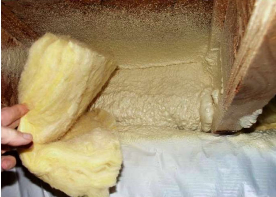
Fix: spray foam or foam block sealed in place. Note: the energy code requires rim/band joist must have an air barrier.
