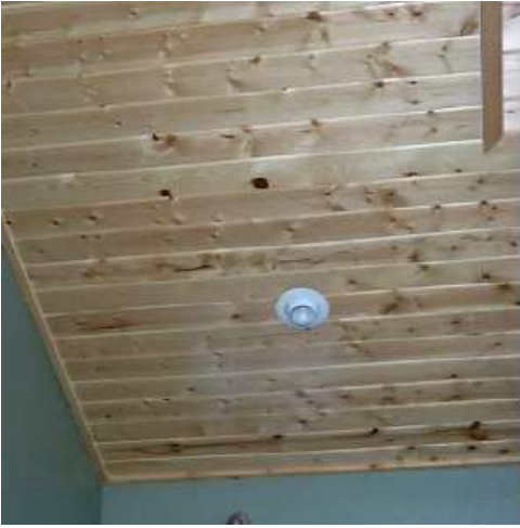
Recessed lights and unsealed wall ceiling junction.
