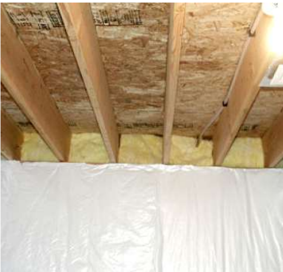
Rim/band joist of crawl spaces, basements and between floor. Note: fiberglass is not an air barrier, it does not stop air flow.
