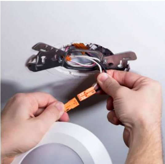
Fix: seal standard box from the attic or install air tight boxes and LED lights. LED surface mounted light fixture with an air sealed electrical box.
