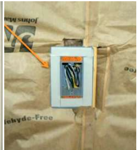
Fix: seal (caulk) sides of electrical box to sheetrock (above left and center). Fix: wide flange, with sealed (foamed in place) wiring opening boxes, compressed foam gasket seals box to wall board (above right).
