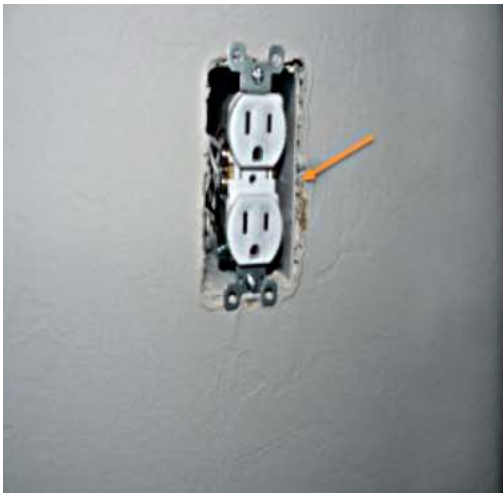
Fix: seal (caulk) sides of electrical box to sheetrock (above left and center). Fix: wide flange, with sealed (foamed in place) wiring opening boxes, compressed foam gasket seals box to wall board (above right).
