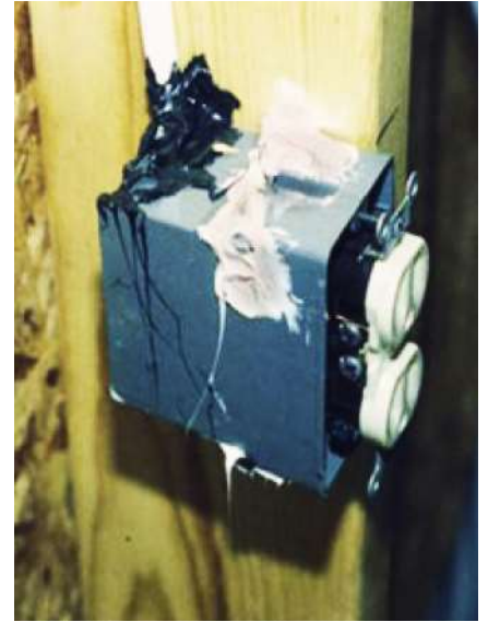
Fix: seal openings in standard box.
